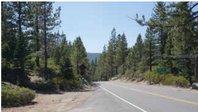
The highway makes an almost 90 degree bend as it enters Meeks Bay which reduces the sight distance for pedestrians crossing the road.
