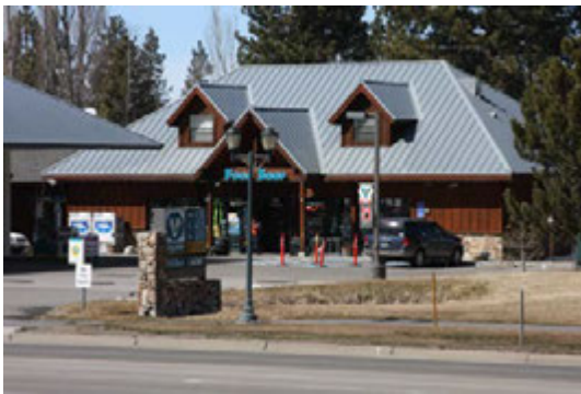
Valero Gas Station Rebuild
