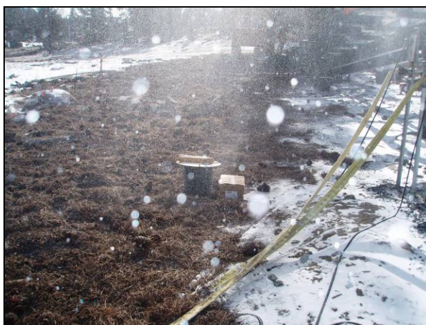
Figure 28. Tubing lift, access road winterized with wood chips (tilled) and pine needle mulch after construction, December 2010.
