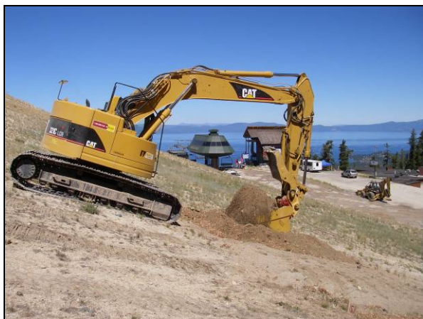
Figure 3. Tilling/scalloping with full-sized excavator
