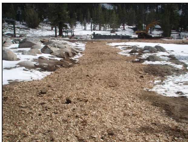
Figure 27. Tubing lift, snowmaking lateral covered in wood chips during construction, treatment area A, October 2009.
