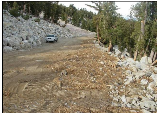
Figure 115. Infiltration strip and rock slope protection in lower segment of Skyline Trail.
