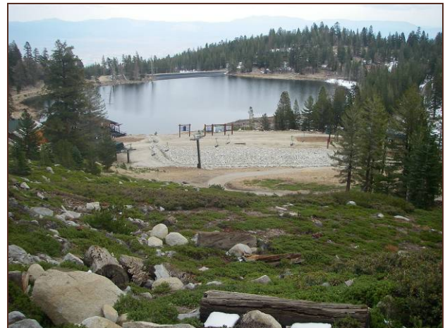
Figure 113. Skyline Trail Dipper bottom slope, after rock application, 2009.
