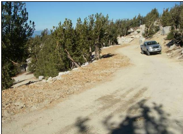
Figure 114. Infiltration strip in upper segment of Skyline Trail.
