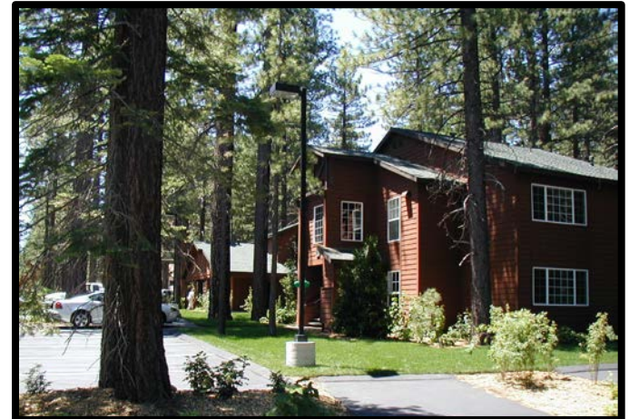
Evergreen Tahoe Apartments, South Lake Tahoe, CA
