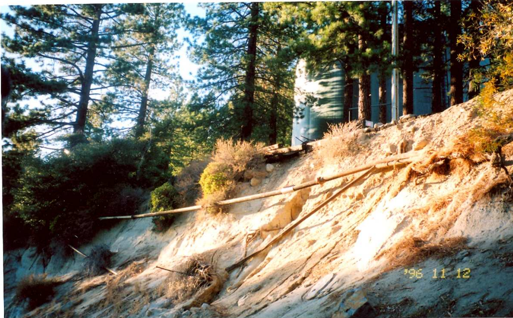
Photo No.: 1 Date: 11/20/08 Time: 3:30pm Description: overview of parallel pipelines; six-inch line (top), four-inch line (bottom and broken); note steep and eroded cut bank; modern water tank on Reservoir Drive (back right); view is 265°
