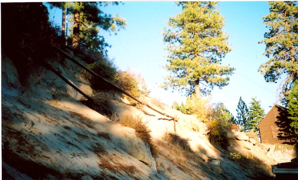
Photo No.: 2 Date: 11/20/08 Time: 3:30pm Description: overview of parallel pipelines; six-inch line (top), four-inch line (bottom); note steep and eroded cut bank; ca. 1910s building (bottom right); view is 50°
